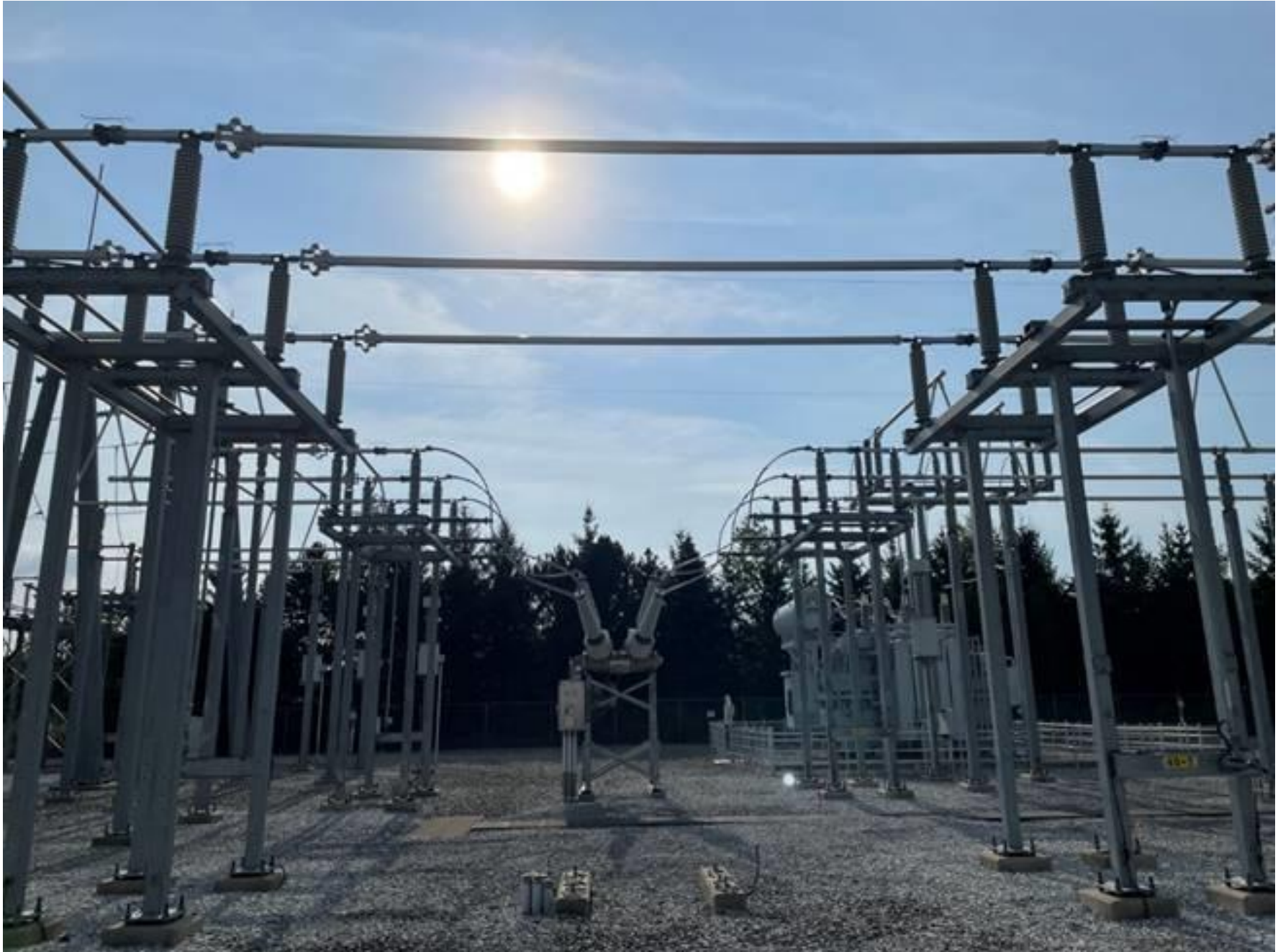
Future breaker position showing installed foundations and conduits
