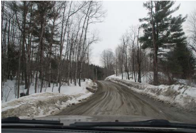
View Headed Southbound on Gregg Hill Road
