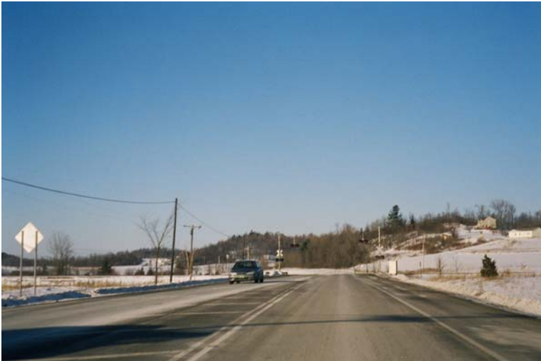
Photo 13 Ferrisburgh Route 7 crossing looking north.
