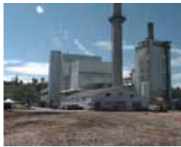
Burlington, VT Wood Plant McNeil Station Credit: Electric Dept.
