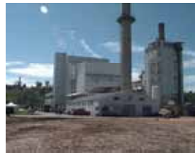
Burlington, VT Wood Plant McNeil Station Credit: Electric Dept.
