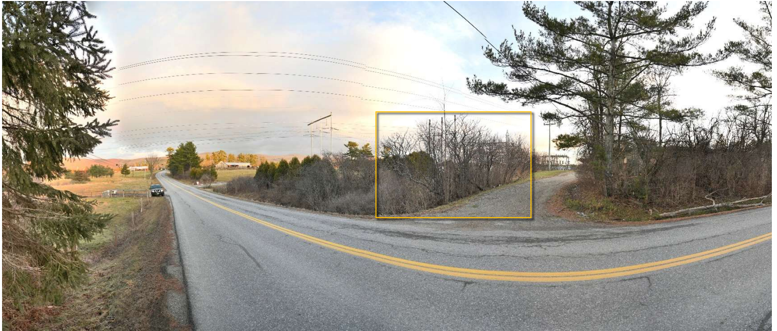
Viewpoint 1: Approximately 180° panoramic view from Quarry Road just northwest of the VELCO Middlebury Substation. This view pans from roughly northeast (left) to southwest (right) and shows the surrounding area along Quarry Road near to the existing Substation. The orange rectangle towards the right of this image represents the following photo, which is captured with a 50mm equivalent lens.
