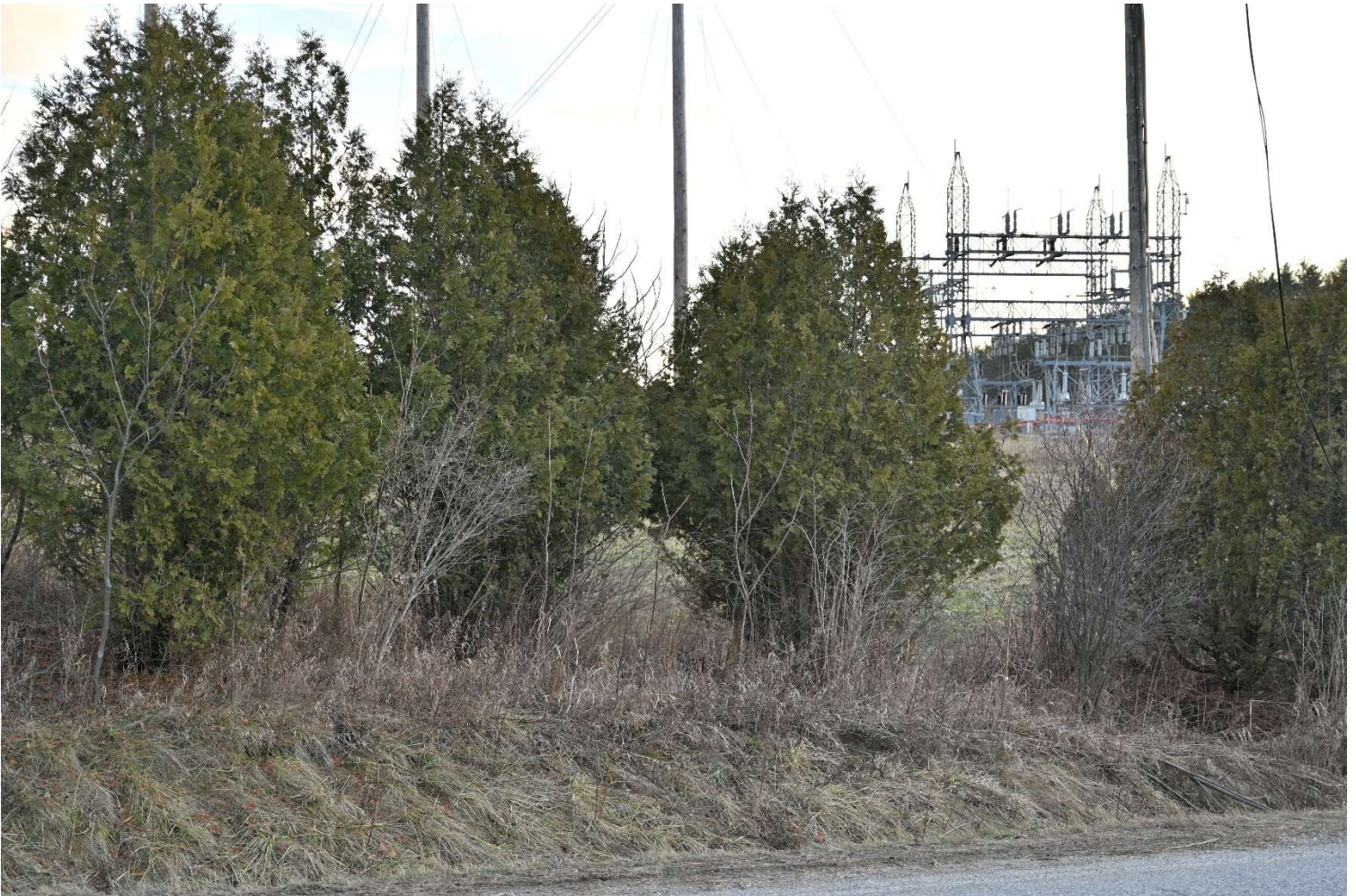
Viewpoint 3: View looking southwest from Quarry Road towards the existing substation and proposed upgrades. This view is represented by the orange rectangle in the image above.
