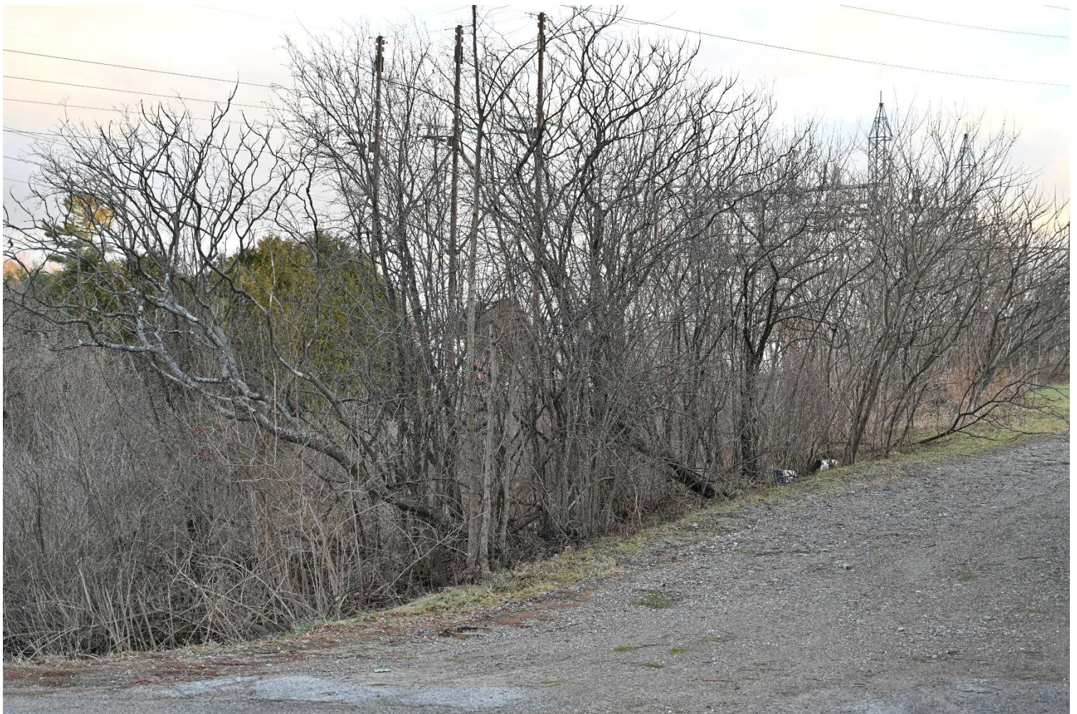
Viewpoint 1: View looking southeast from Quarry Road towards the existing substation and proposed upgrades. This view is represented by the orange rectangle in the image above.
