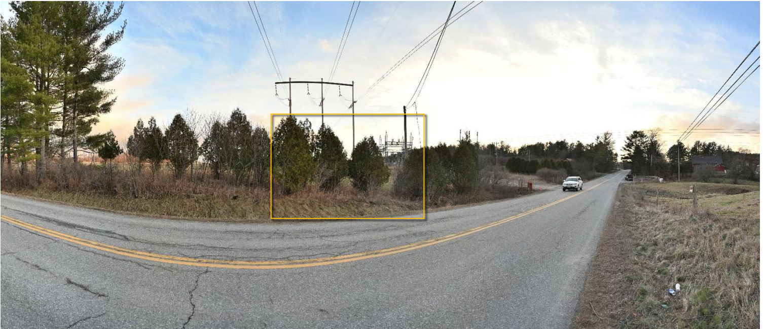
Viewpoint 3: Approximately 180° panoramic view from Quarry Road just northeast of the VELCO Middlebury Substation. This view pans from roughly east (left) to west (right) and shows the surrounding area along Quarry Road near to the existing Substation. The orange rectangle towards the right of this image represents the following photo, which is captured with a 50mm equivalent lens.
