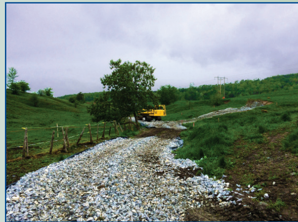
Stone construction access route.
