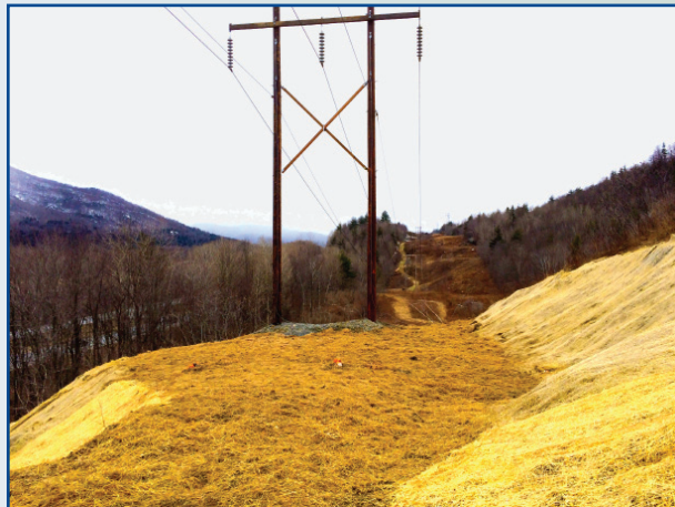
Stabilized work area following structure replacement.
