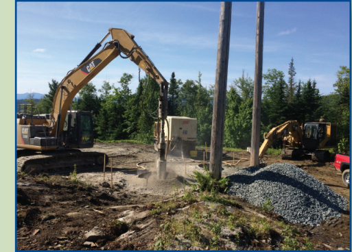
Rock drilling for new pole installation.
