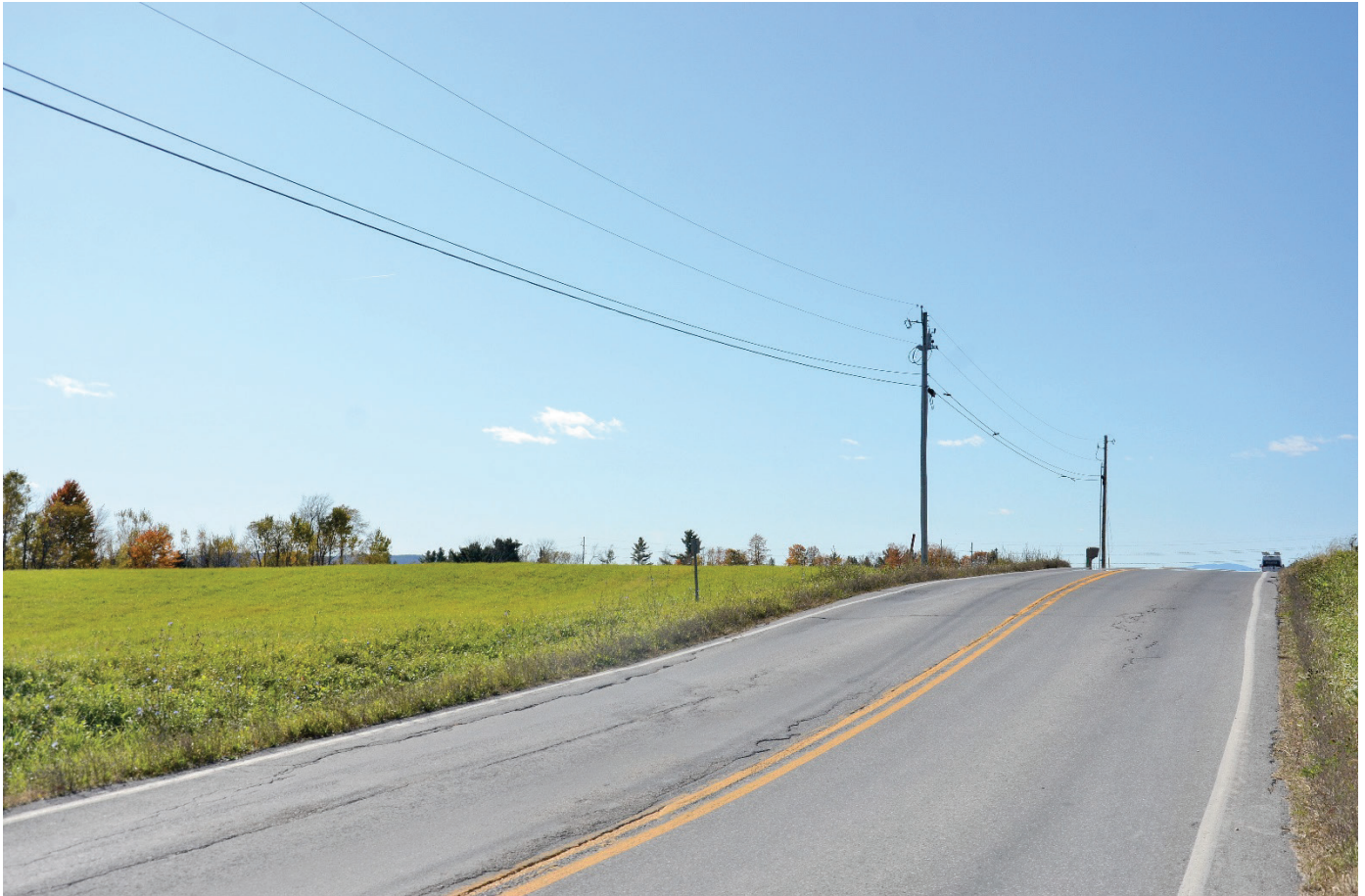
Viewpoint 9: East of the Project site along Vermont Route 17, looking west at existing GMP distribution line.
