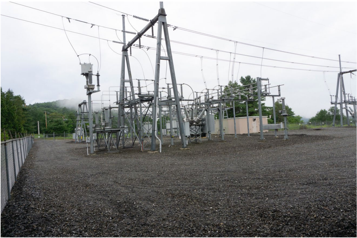
11. 397 Higgins Hill Road looking west
