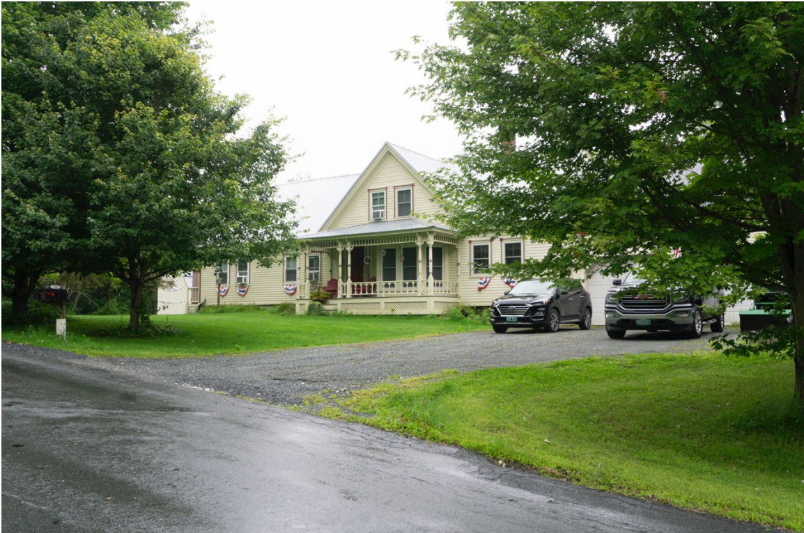
18. 715 Higgins Hill Road looking northwest
