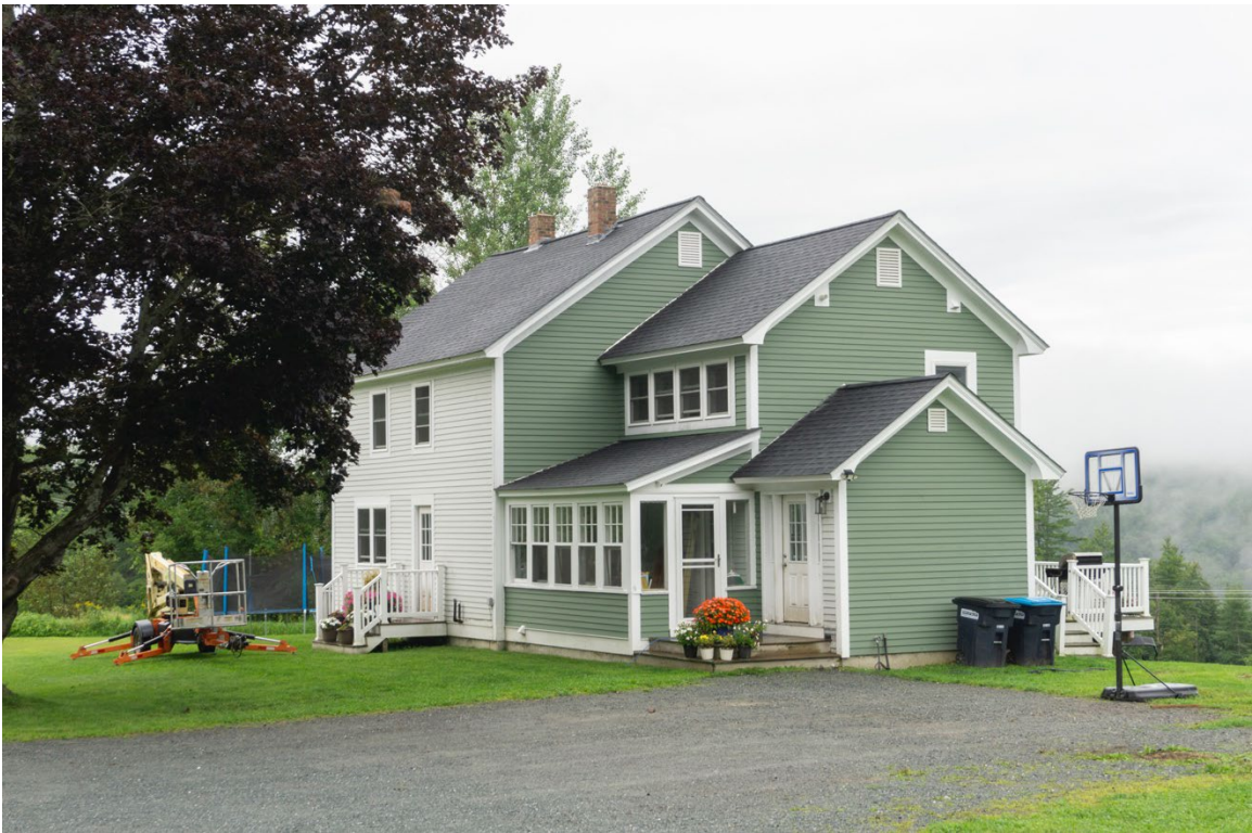
2. 163 Higgins Hill road looking northwest
