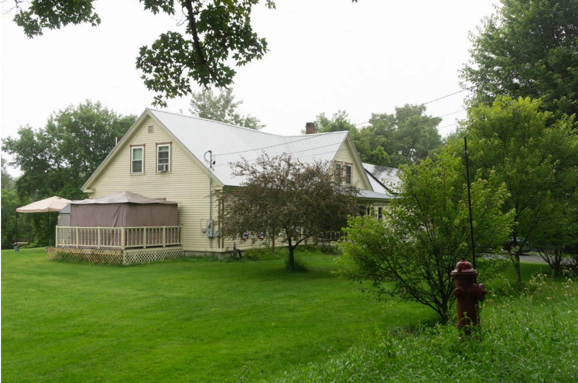
17. 715 Higgins Hill Road looking northeast
