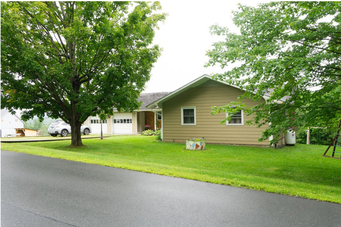
6. 261 Higgins Hill Road looking northwest
