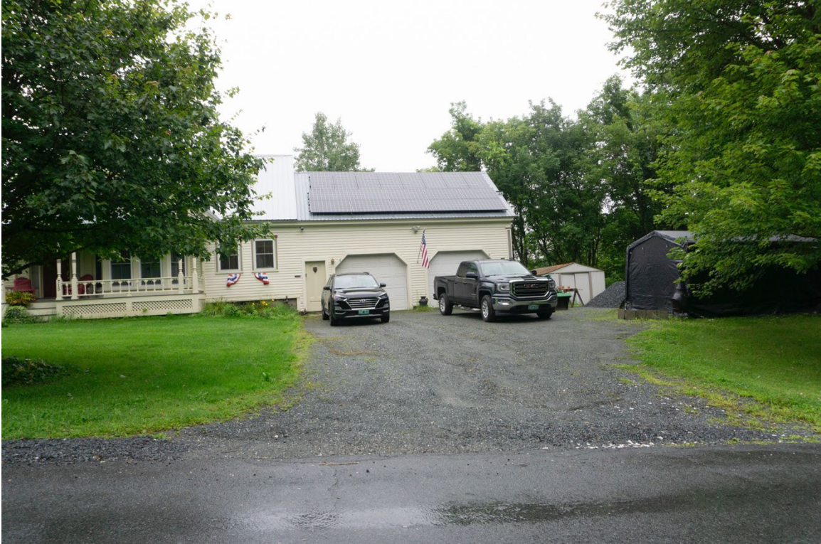
19. 715 Higgins Hill Road garage detail
