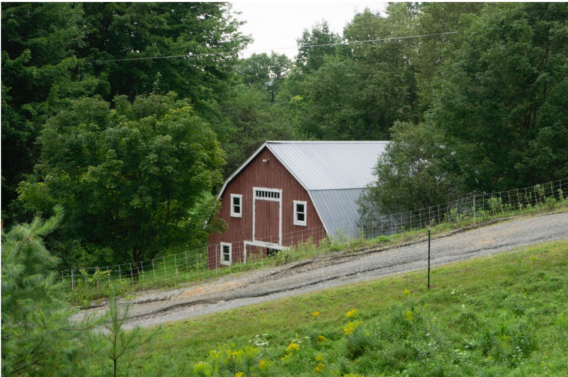
16. 659 Higgins Hill Road looking northeast
