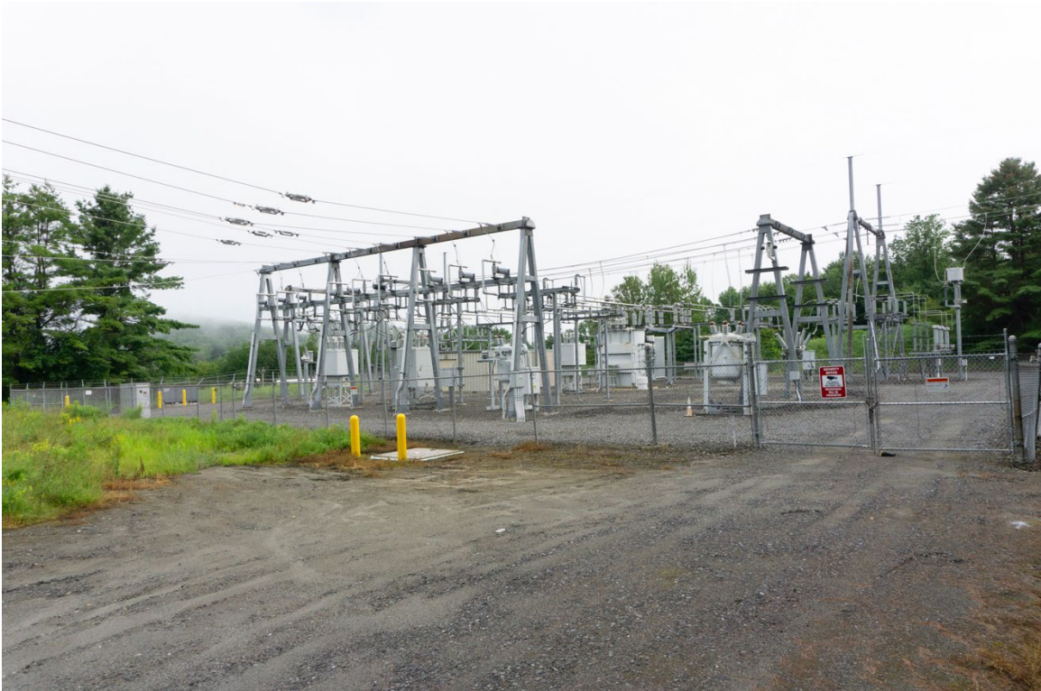
10. 397 Higgins Hill Road looking northeast
