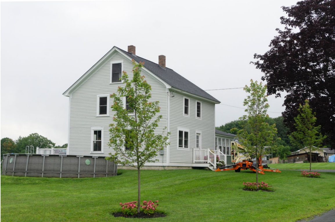
1. 163 Higgins Hill road looking northeast
