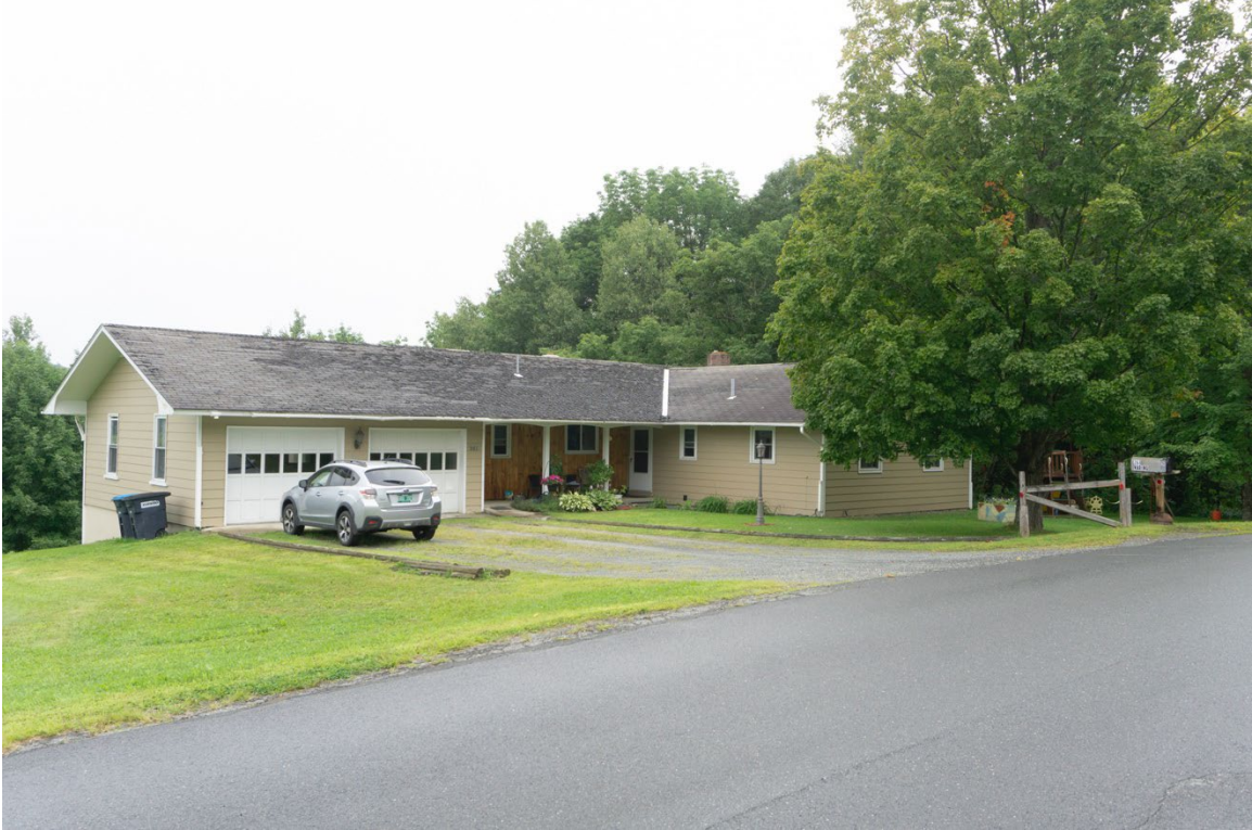
5. 261 Higgins Hill Road looking northeast
