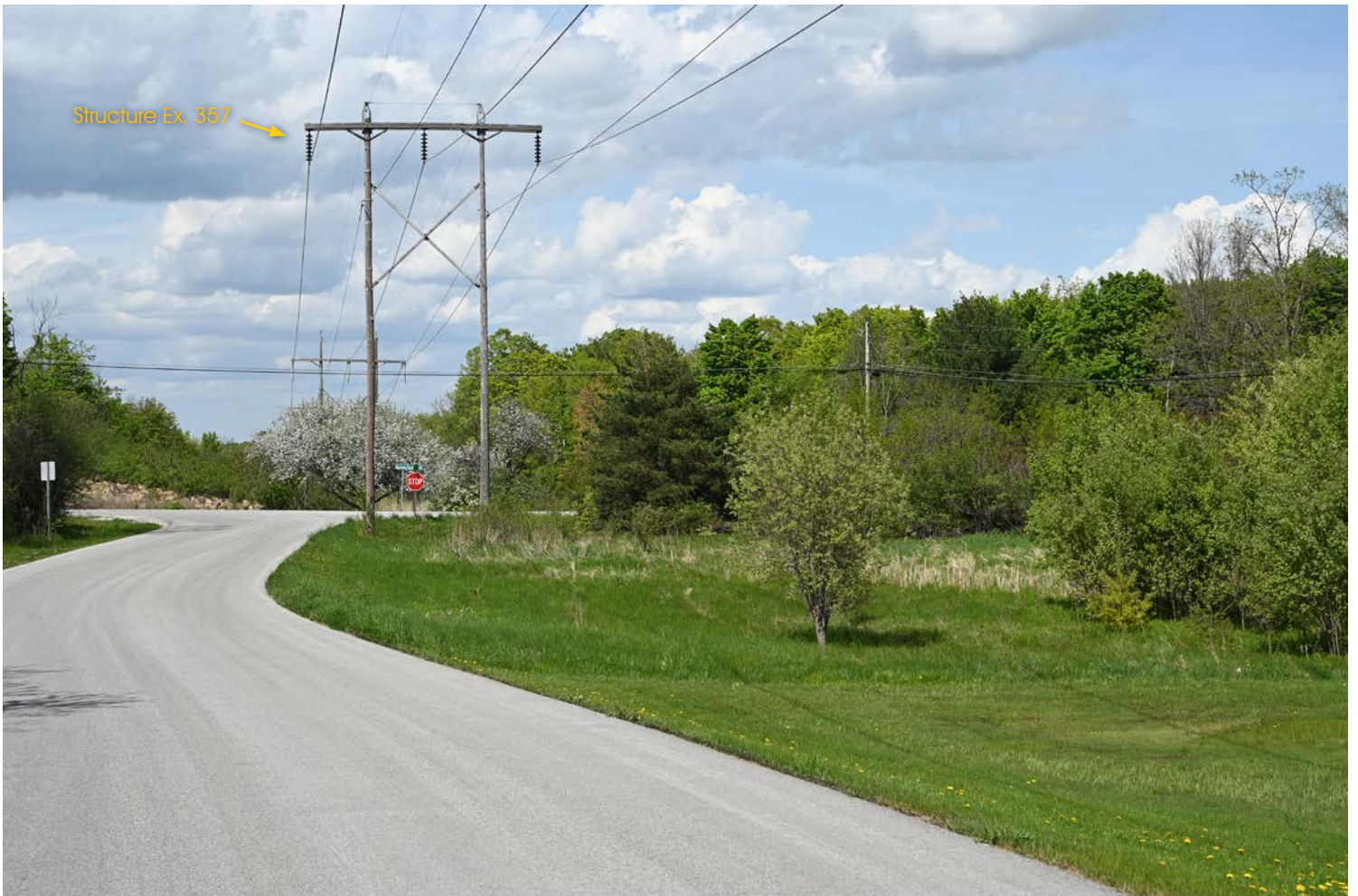
Viewpoint 41: View from Gauthier Drive looking north at structure Ex. 357. (50mm)
