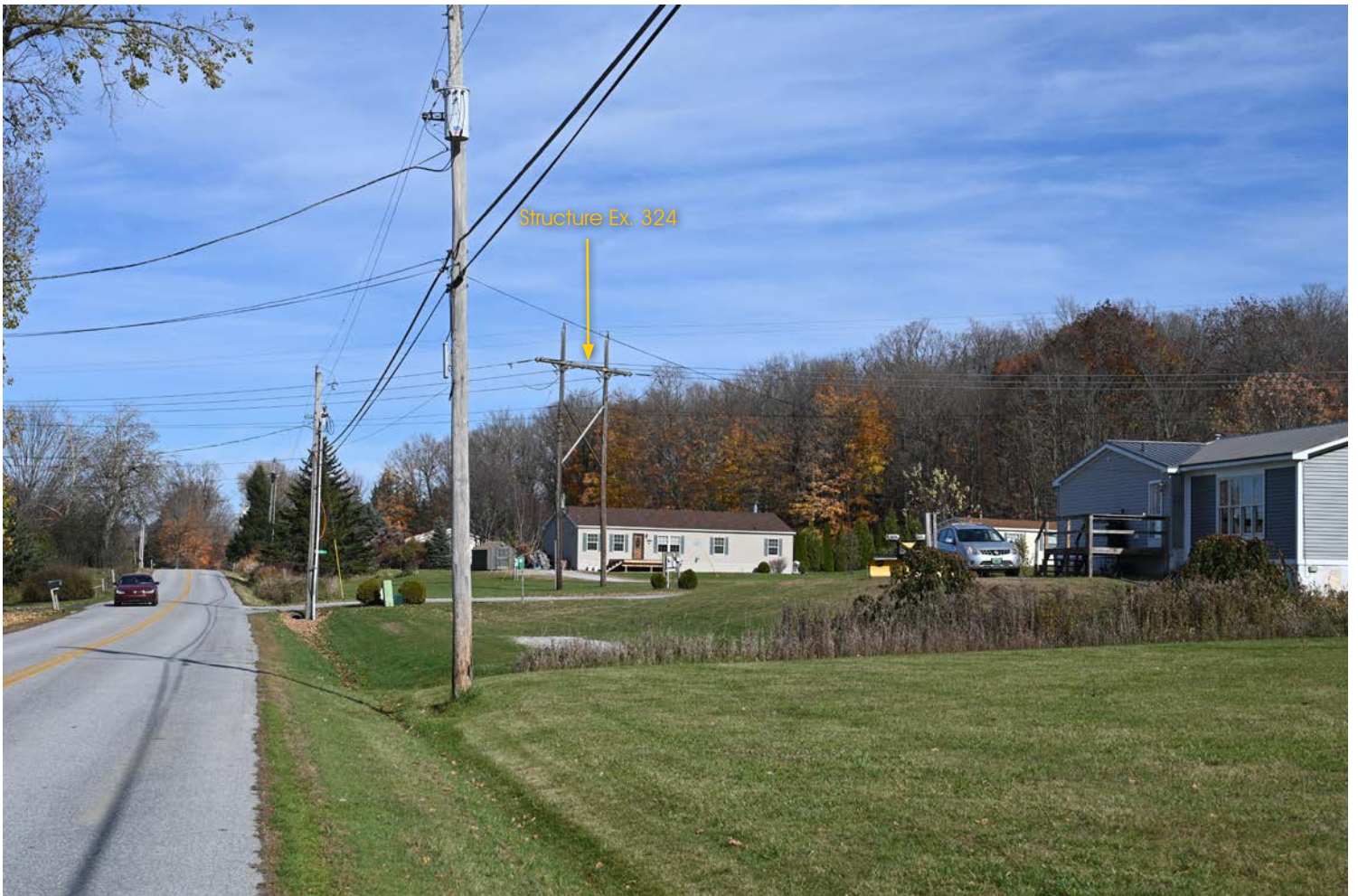
Viewpoint 18: View from Kellogg Road looking northeast towards structure Ex. 324. (50mm)
