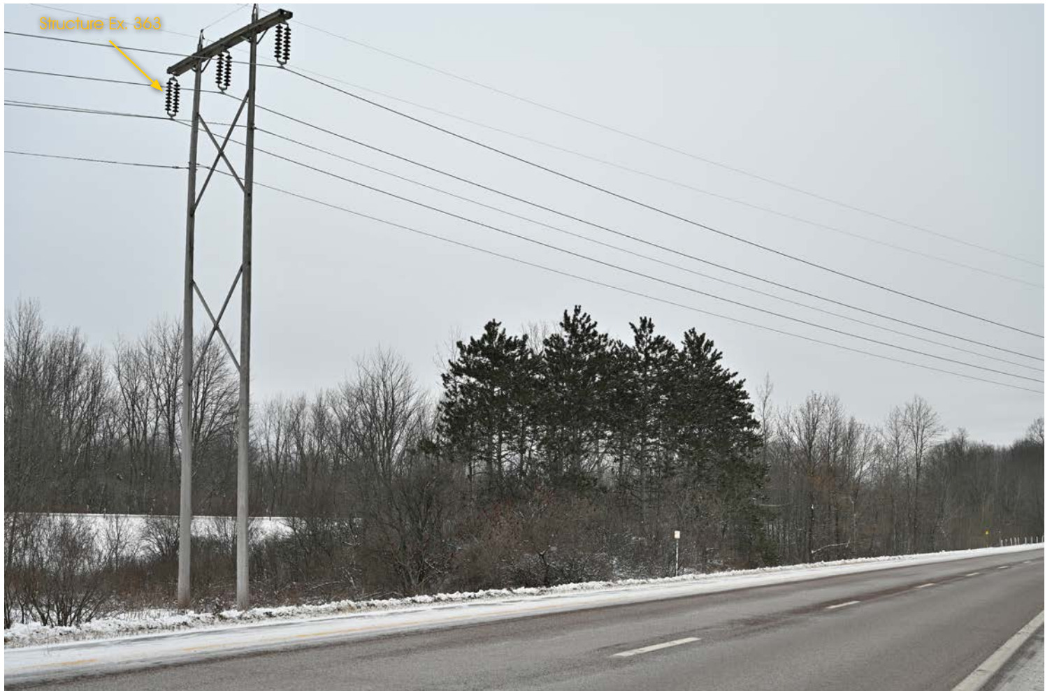
Viewpoint 45: View from I-89 southbound looking southeast (50mm)
