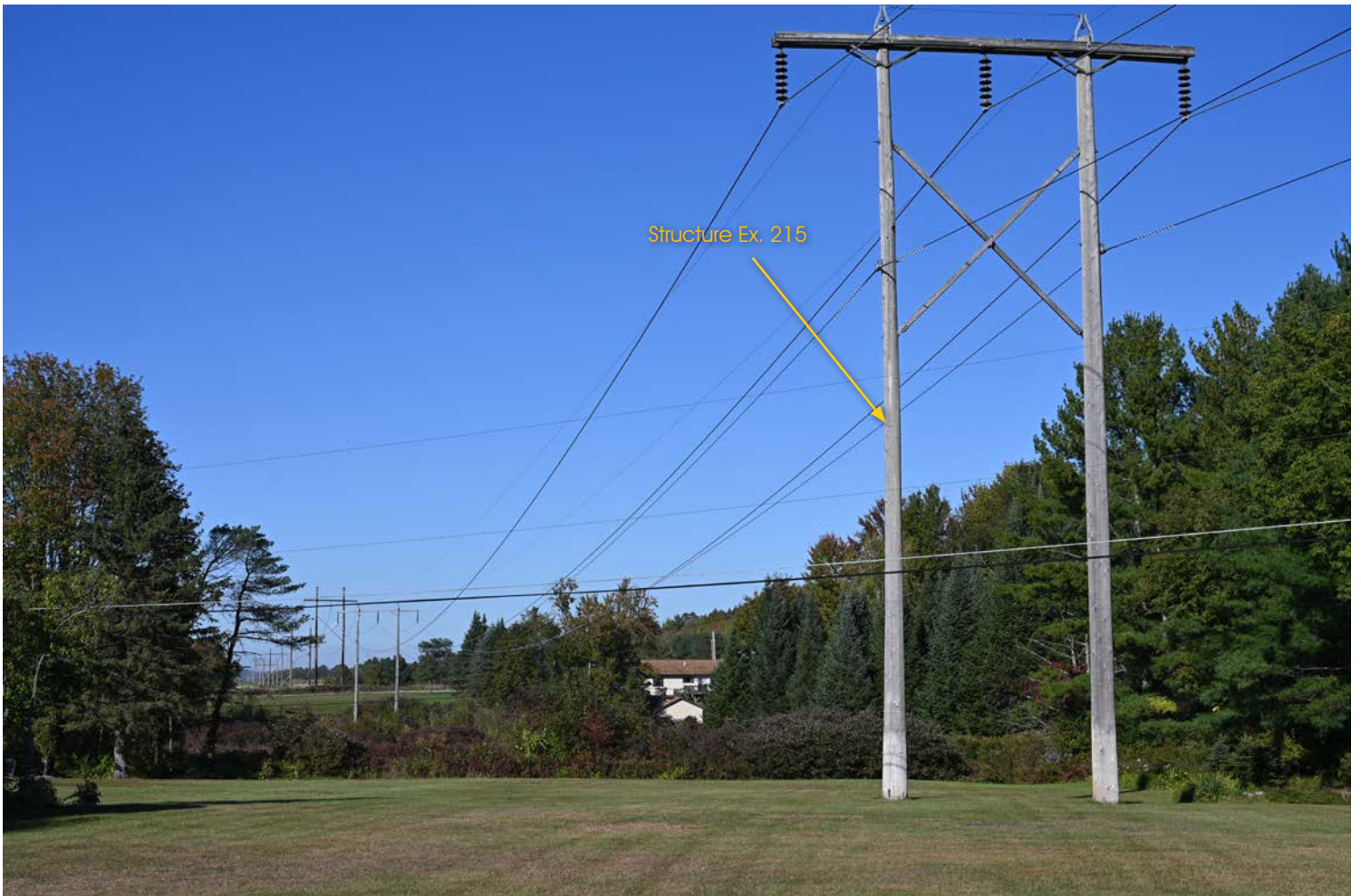
Viewpoint 3: View from Decker Road looking north towards structure Ex. 215. (50mm)
