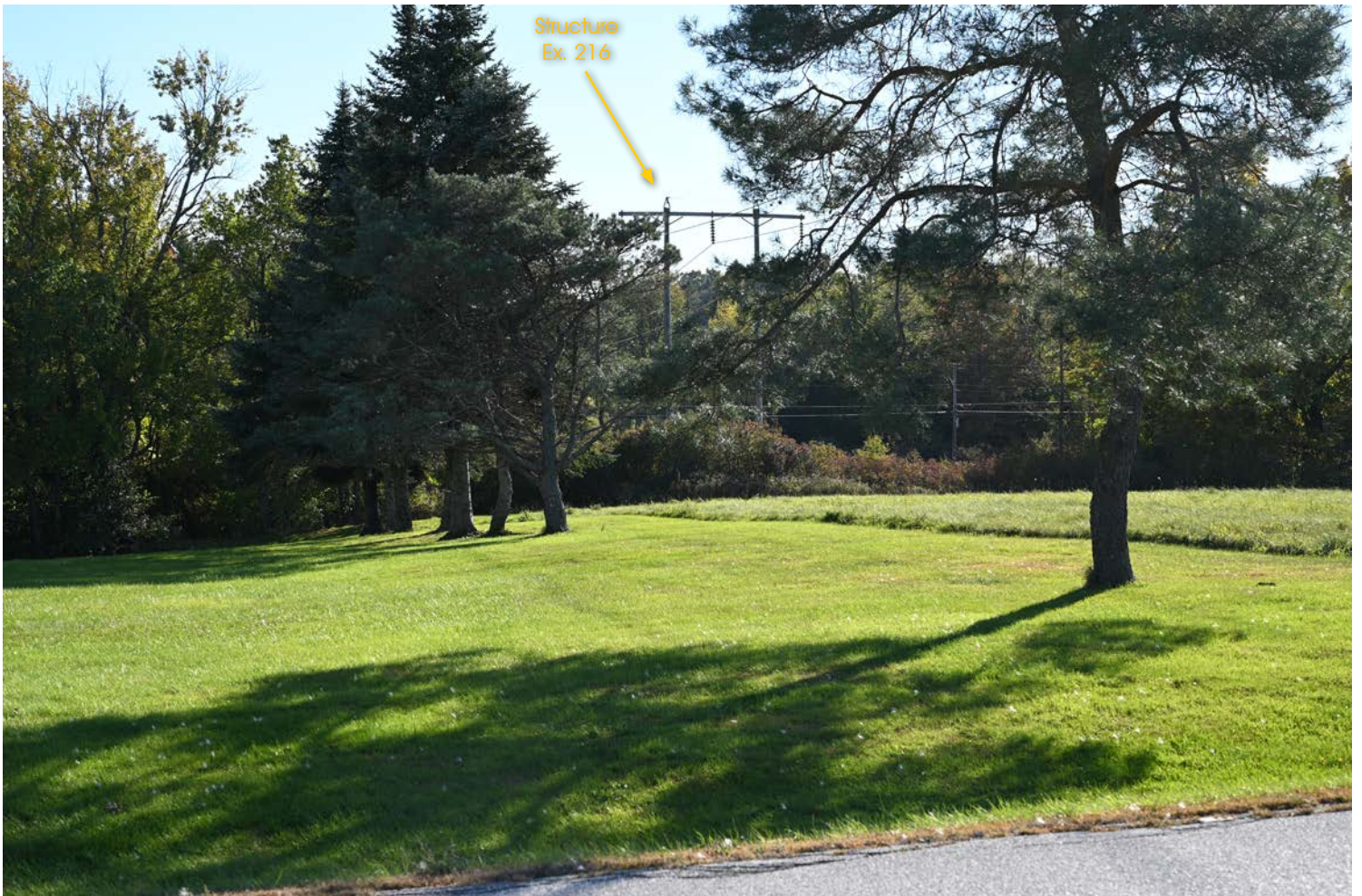
Viewpoint 5: View from Plains Road looking southwest towards structure Ex. 216. (50mm)
