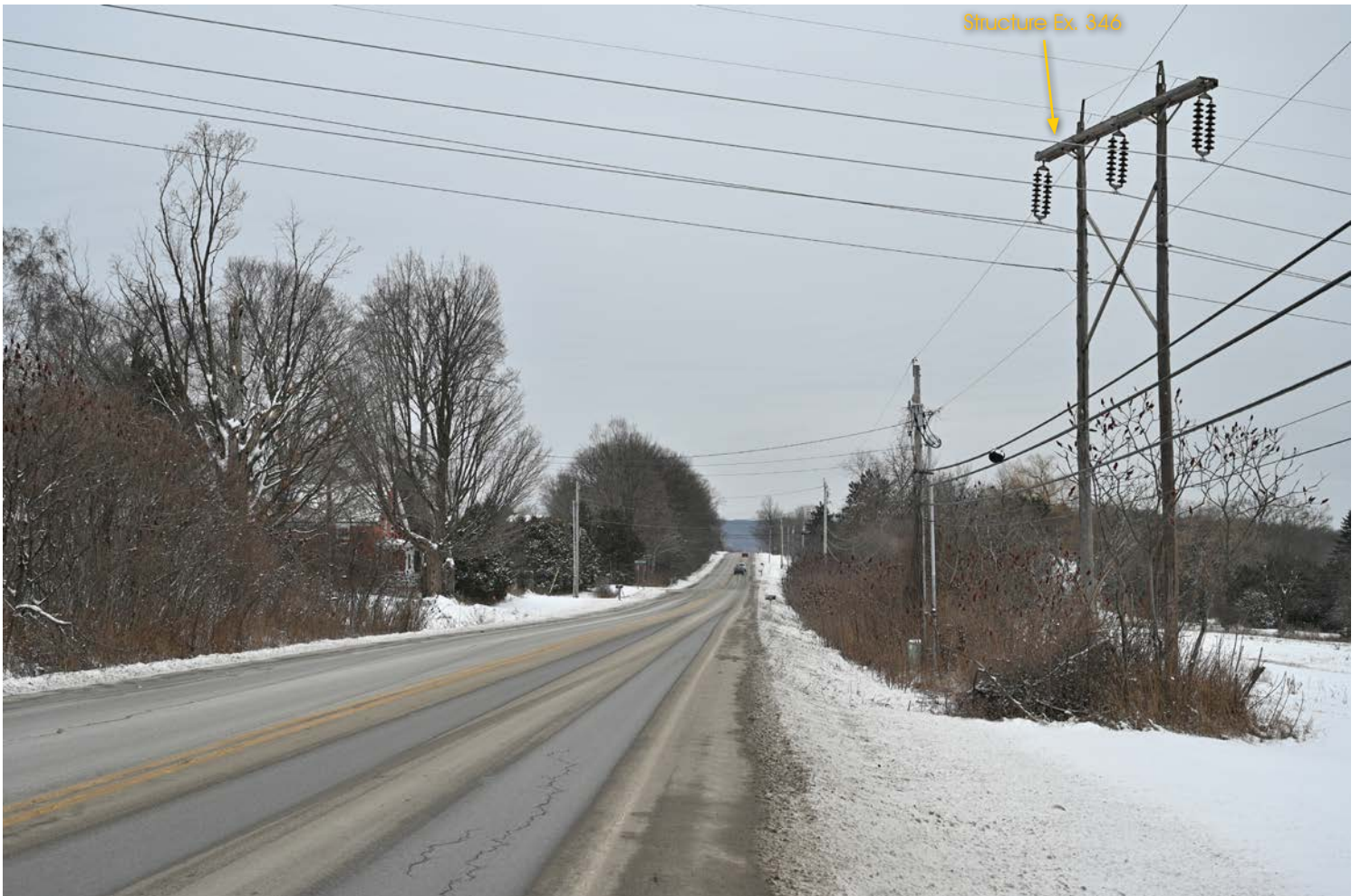
Viewpoint 33: View from St. Albans Road (Route 7) looking south towards structure Ex. 346. (50mm)
