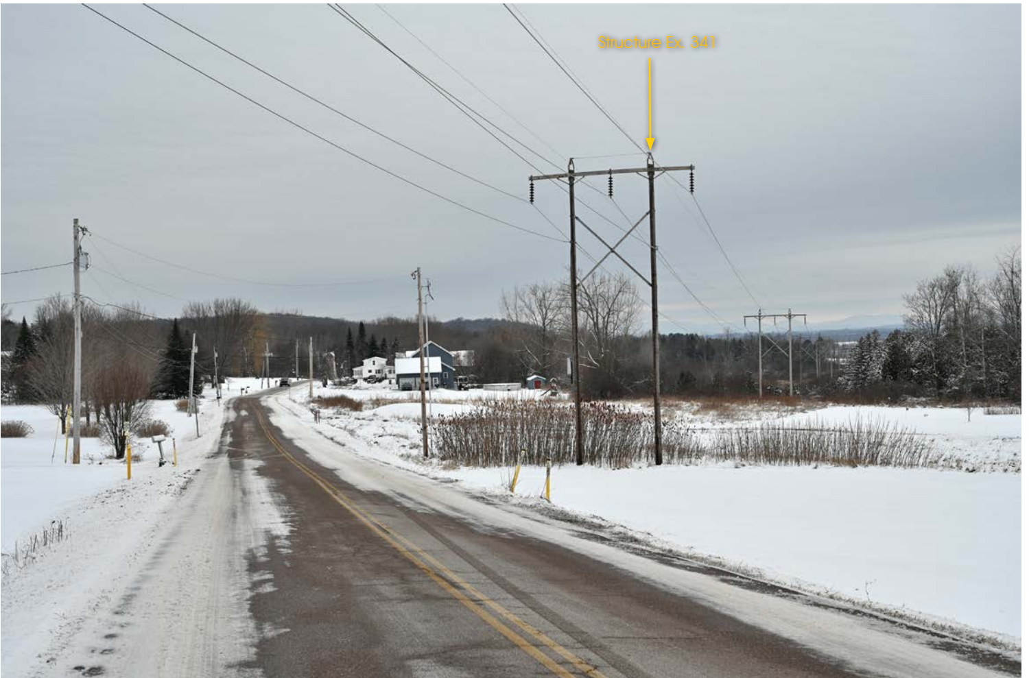
Viewpoint 27: View from Kellogg Road looking southwest towards structure Ex. 341. (50mm)
