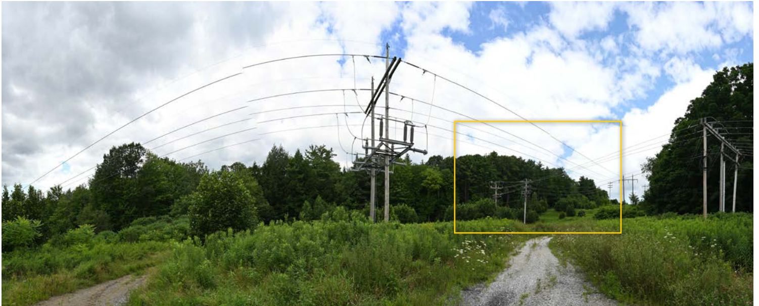
Viewpoint 56: Approximately 180° panoramic view from the Portage Trail, panning from south (left) to north (right). The orange rectangle represents the image below, which is captured with a 50mm lens.
