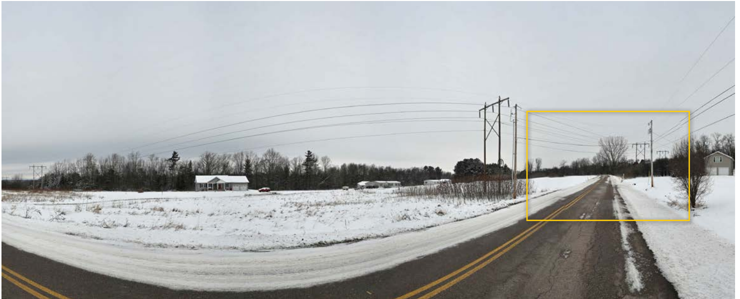
Viewpoint 26: Approximately 180° panoramic view from Kellogg Road, panning from southwest (left) to northeast (right). The orange rectangle represents the image below, which is captured with a 50mm lens.
