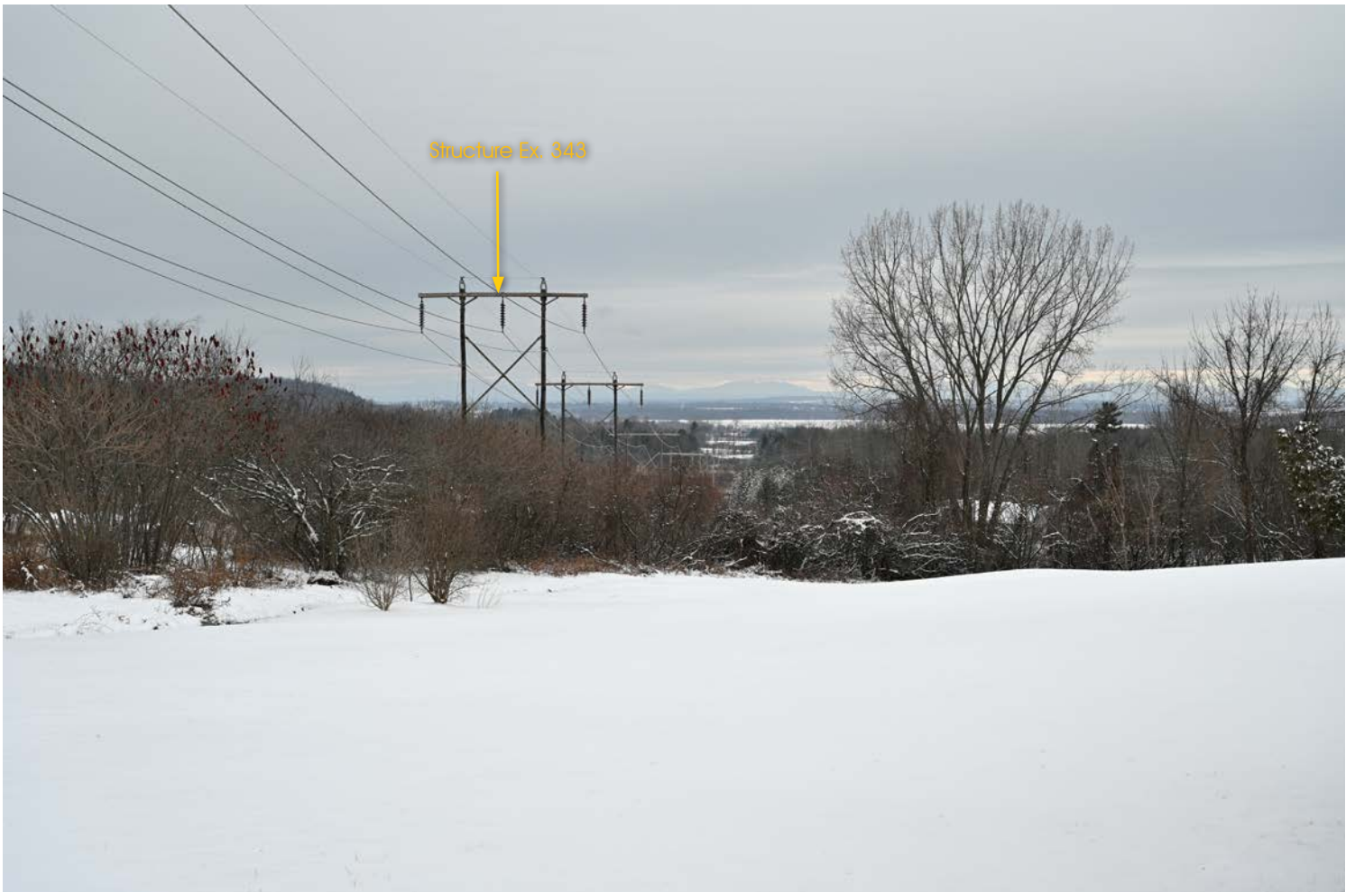
Viewpoint 30: View from Mountain View Drive looking southwest towards structure Ex. 343. (50mm)
