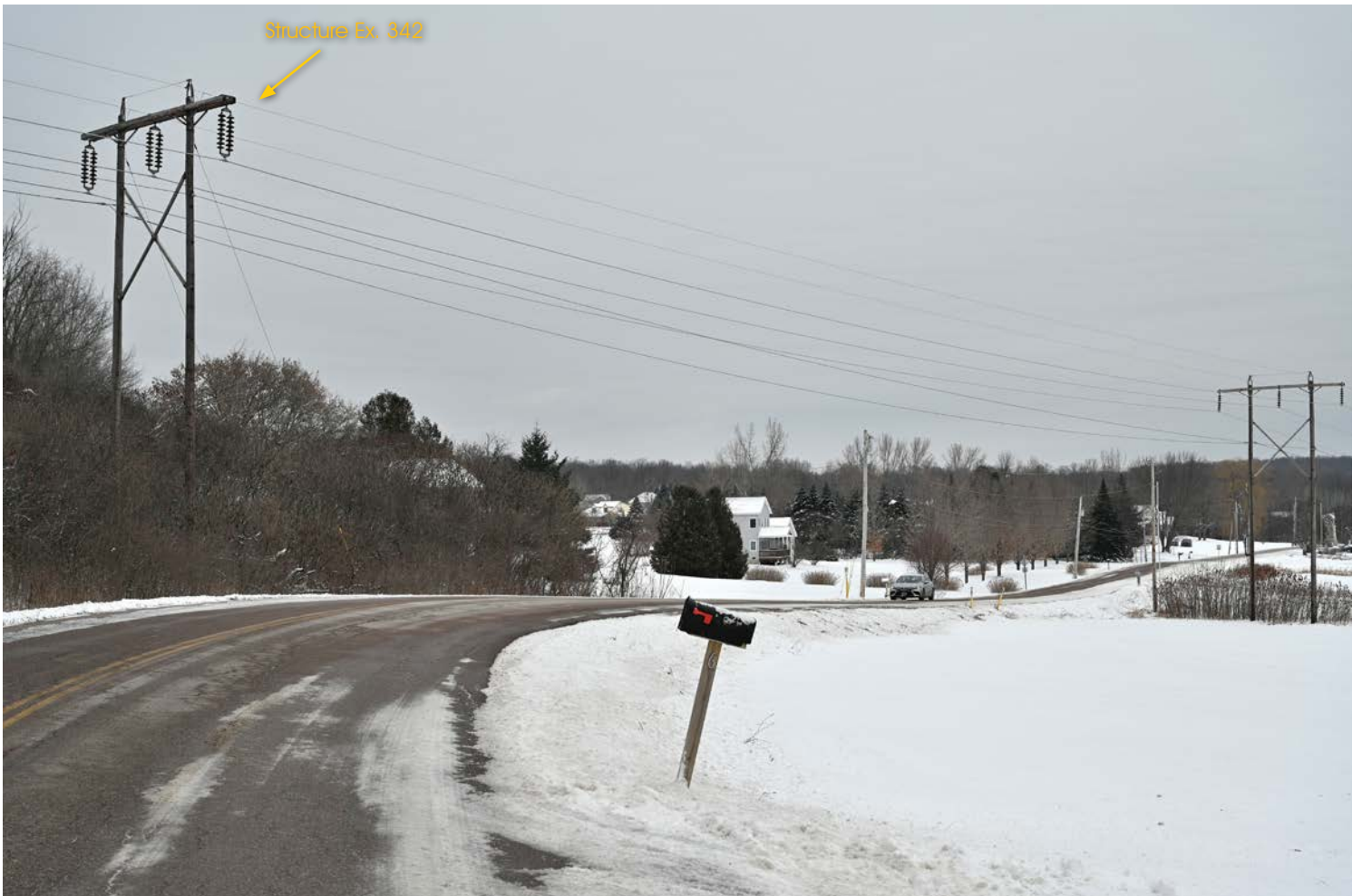
Viewpoint 28: View from Kellogg Road looking south towards structure Ex. 342 (50mm)
