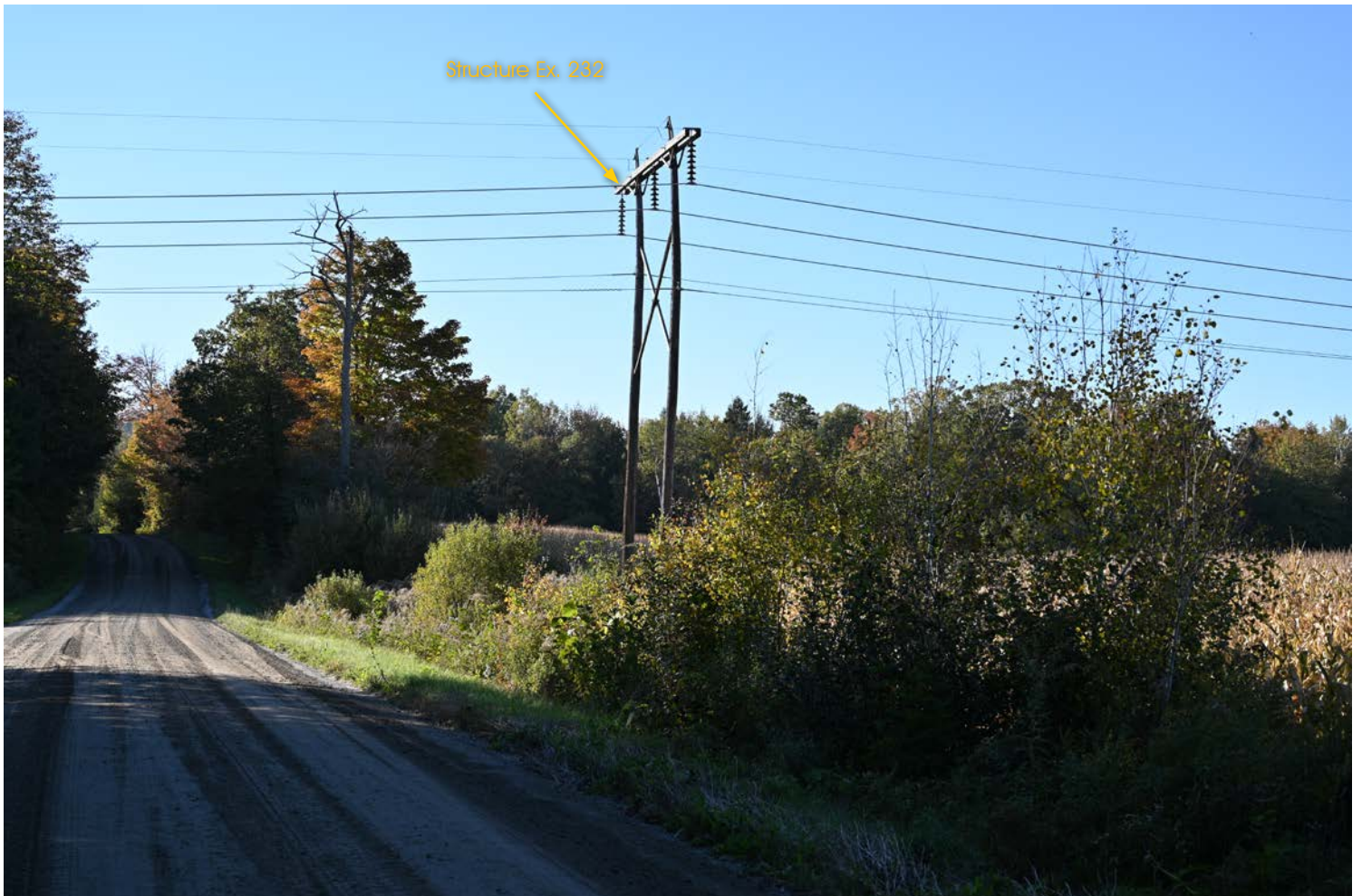
Viewpoint 7: View from Reynolds Road looking northwest towards structure Ex. 232. (50mm)
