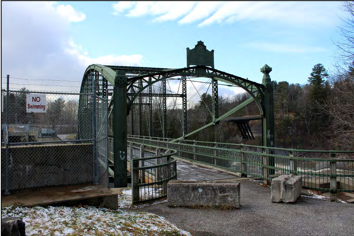
PLATE 6: Douglas & Jarvis Patent Parabolic Truss Iron Bridge, Crossing the Missisquoi River, Looking West
