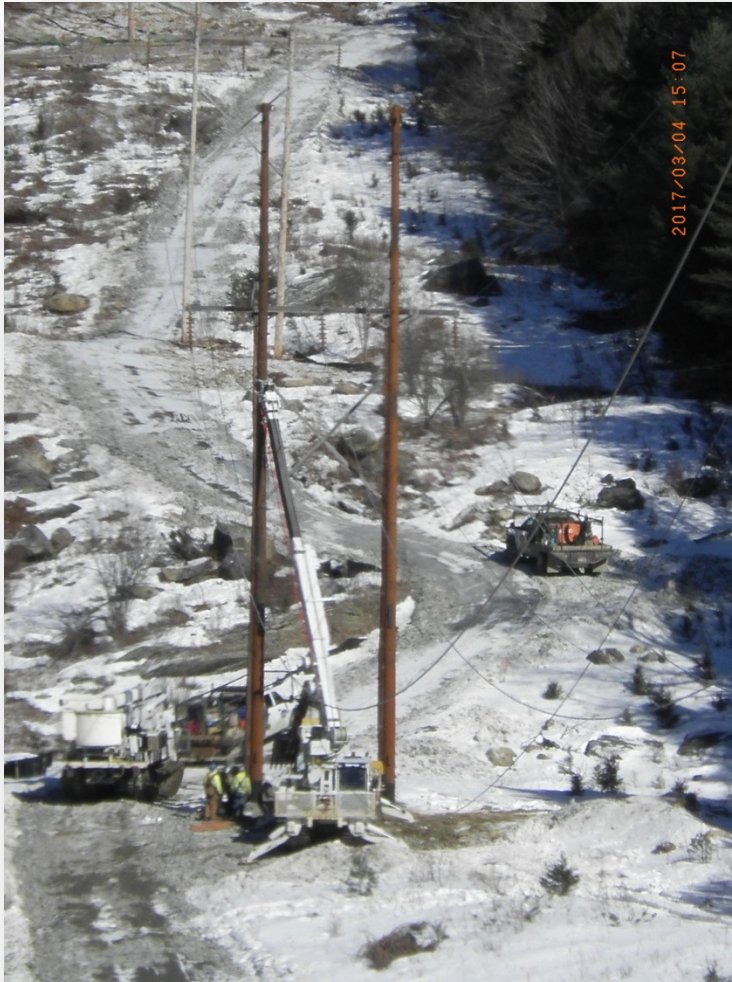
Backfilling and Framing
