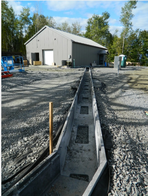
New control building and trench at Barre substation
