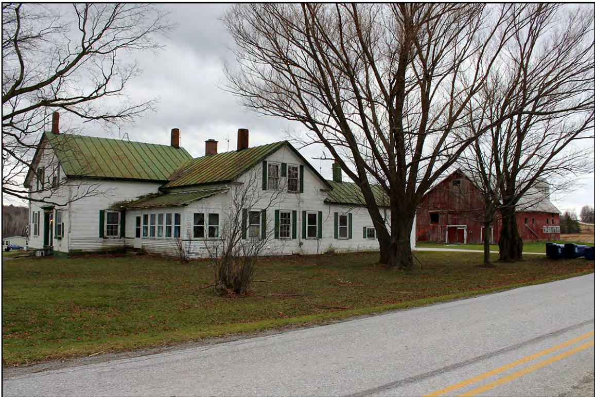
PLATE 19: Jennison-Hubbard Farm and Barn, 2162 Highgate Road, Swanton, Looking Southwest
