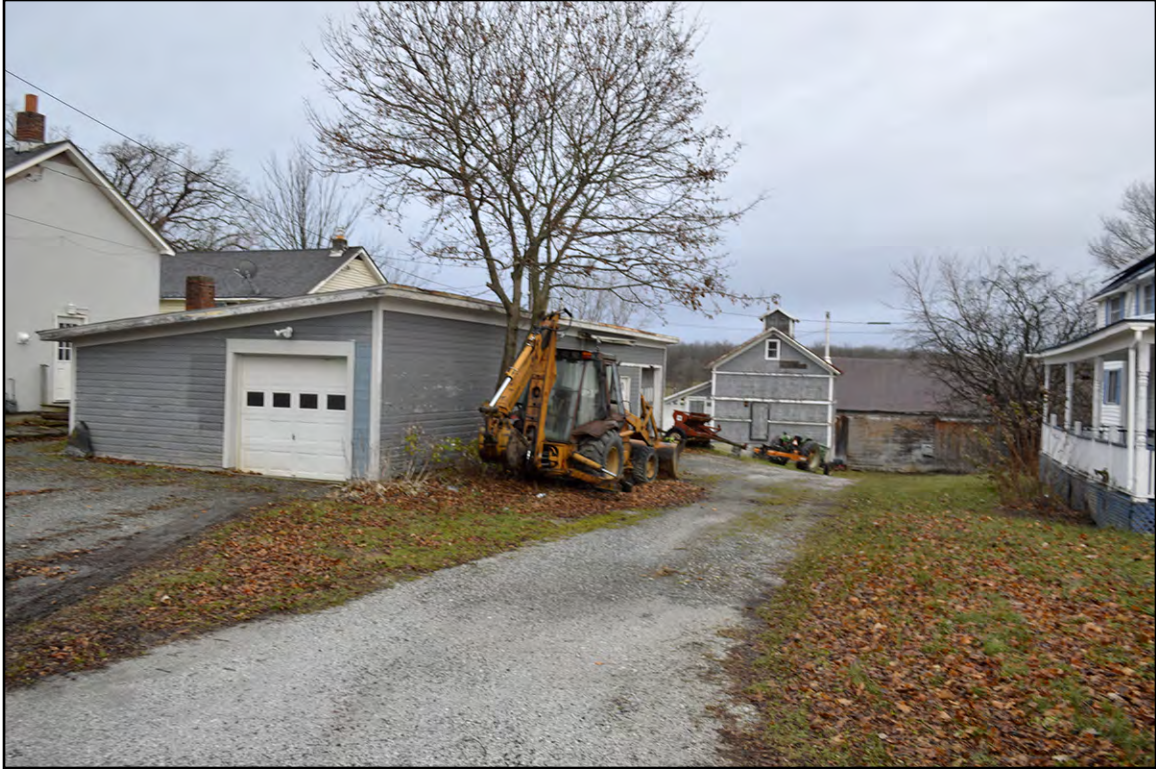
PLATE 35: Brigham-Lareau Farm Barn, 129 Brigham Road, St. Albans, Looking West
