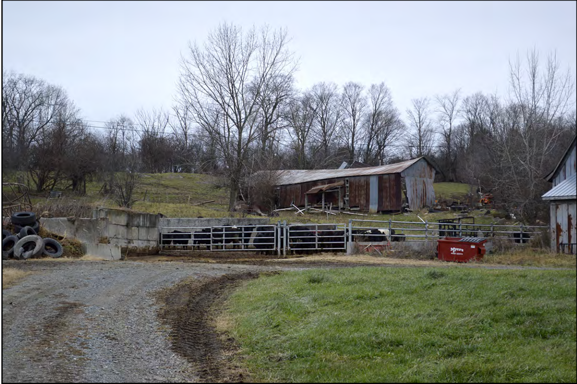
PLATE 83: Cattle Pen and Barn at Sabin-Nye House, 586 Plains Road, Georgia, Looking Northwest
