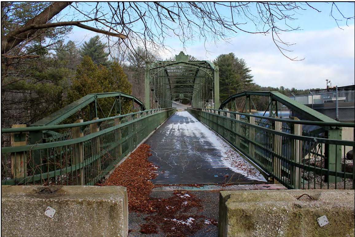
PLATE 7: Douglas & Jarvis Patent Parabolic Truss Iron Bridge, Crossing the Missisquoi River, Looking East-Northeast
