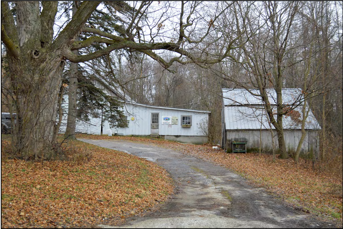
PLATE 33: Barns at Tullar-Dunsmore Farm, 2764 Kellogg Road, St. Albans, Looking East-Southeast
