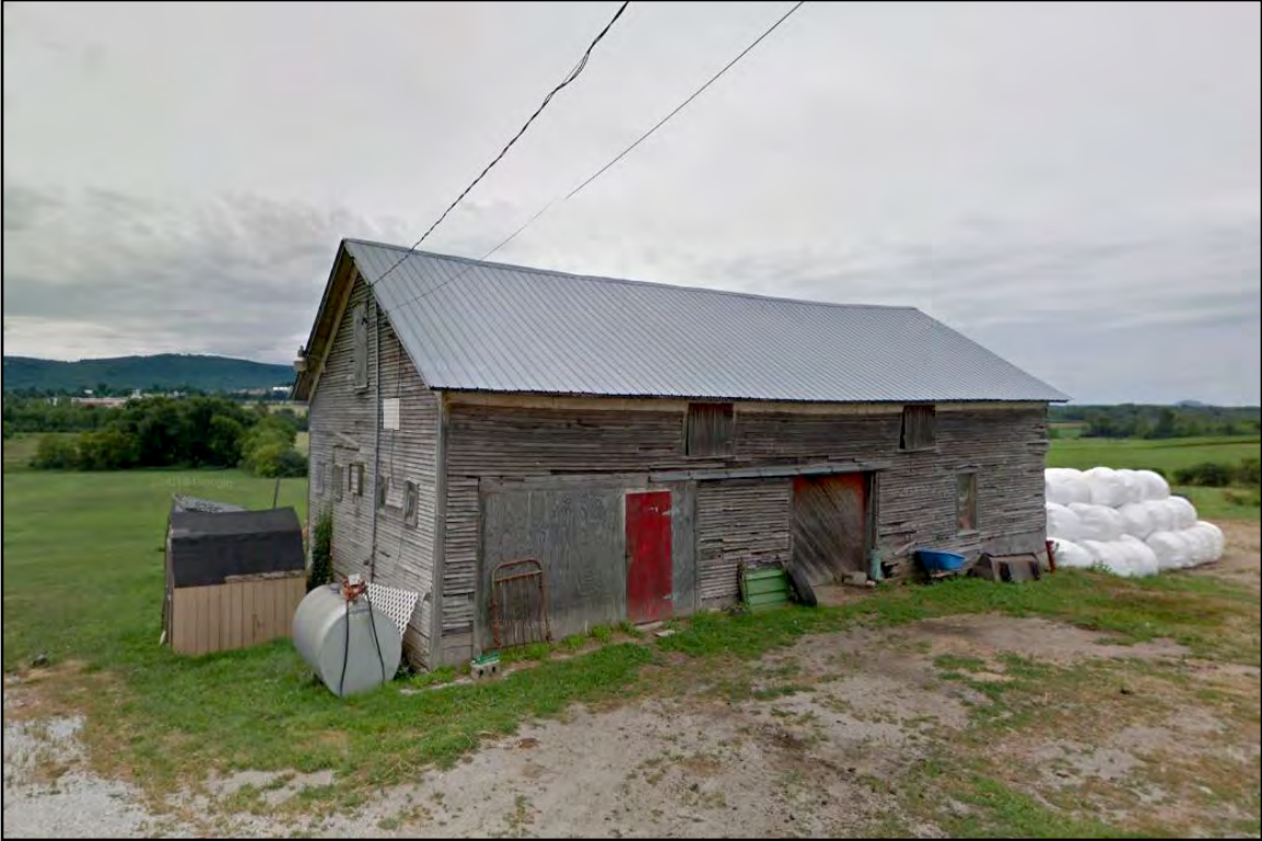
PLATE 48: Barn at Connors-Cameron House, 1715 Bronson Road, St. Albans, Looking Southeast
