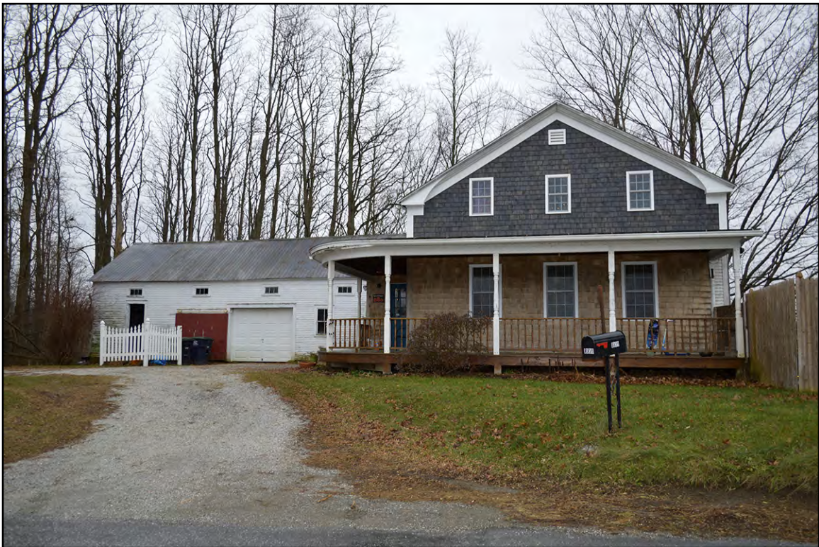
PLATE 60: Meigs-Armstrong House, 1039 Mill River Road, Georgia, Looking South
