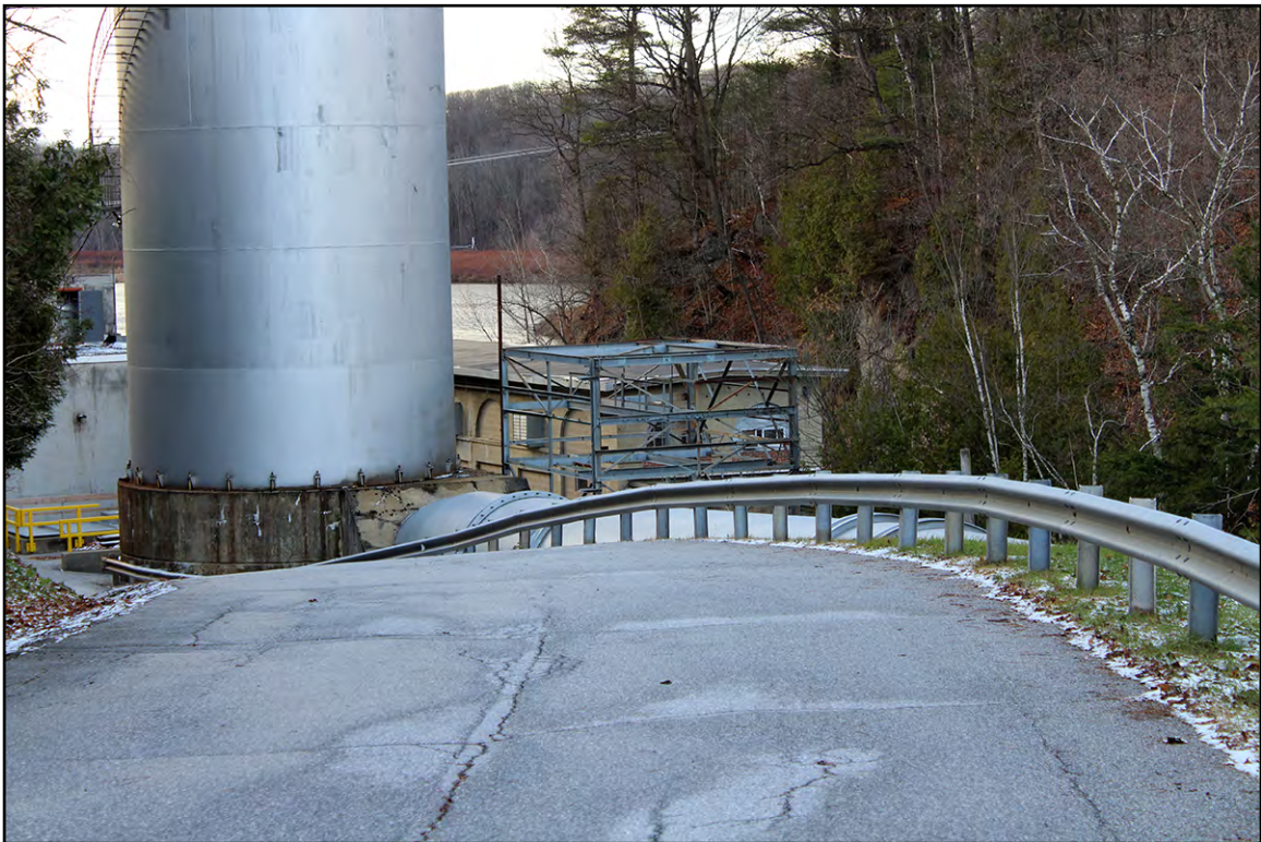
PLATE 3: Highgate Falls Power Plant, Baker Road Along the Missisquoi River, Looking Southwest
