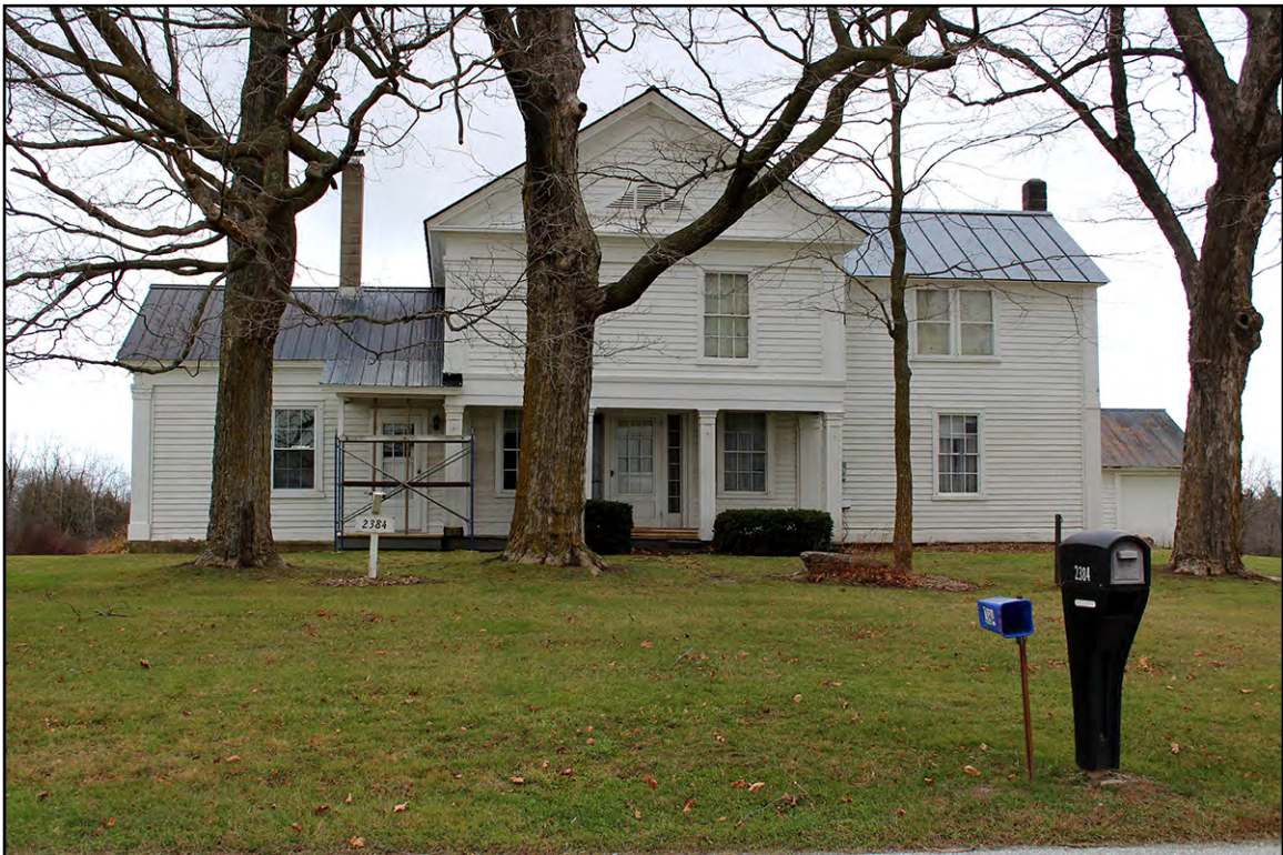
PLATE 13: Tarte House, 2384 Highgate Road, Swanton, Looking West-Northwest
