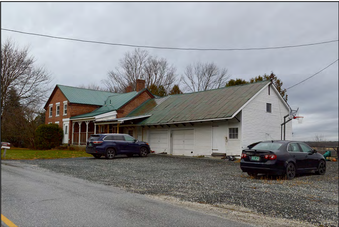
PLATE 30: Brooks-Larson Farm, 2331 Kellogg Road, St. Albans, Looking Southwest
