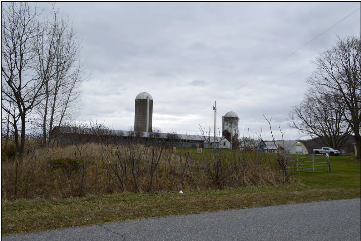
PLATE 58: Outbuildings at Georgia Poor Farm, 846 Mill River Road, Georgia, Looking Northeast
