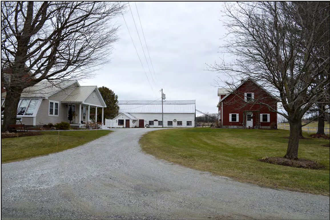
PLATE 76: Barn and Carriage House at Parent Farm, 854 Pattee Hill Road, Georgia, Looking North
