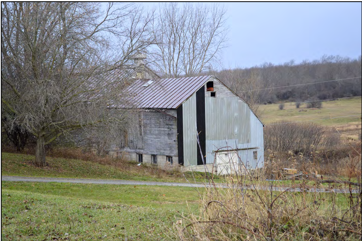
PLATE 36: Brigham-Lareau Farm Barn, 129 Brigham Road, St. Albans, Looking Southwest
