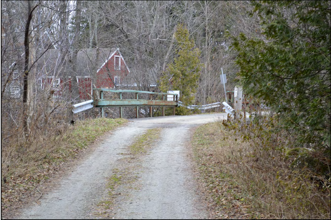
PLATE 61: Pony Truss Bridge, Falls Road over Mill River, Georgia, Looking North
