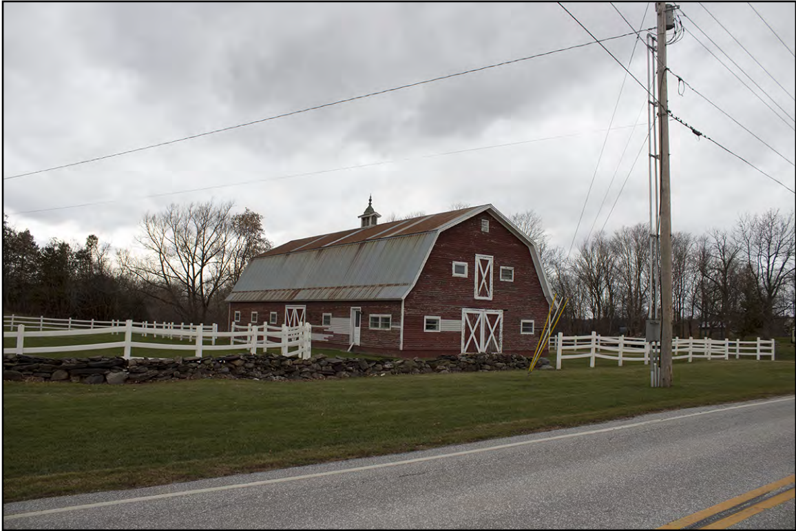
PLATE 10: Barn at Rockledge Farm, 2396 Highgate Road, Swanton, Looking Northwest
