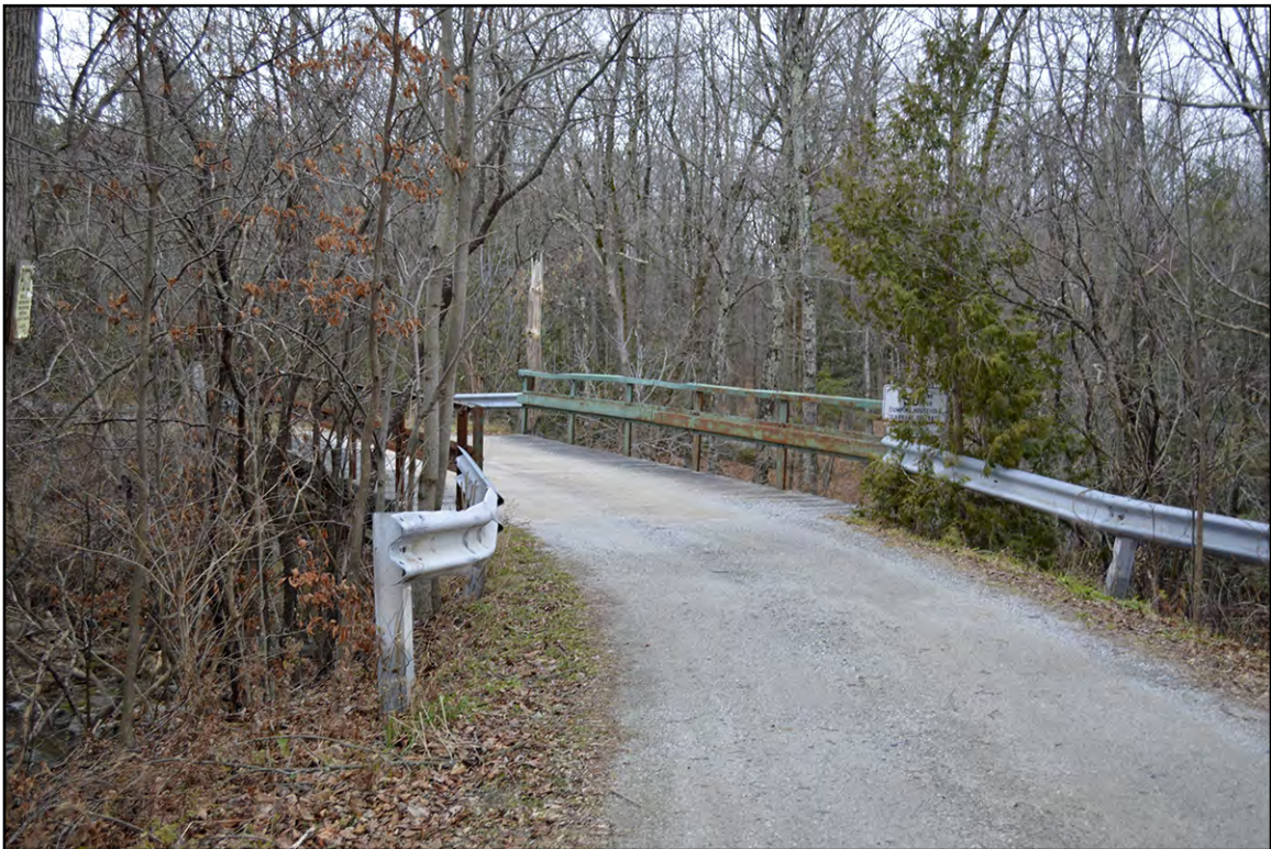
PLATE 62: Pony Truss Bridge, Falls Road over Mill River, Georgia, Looking West-Southwest
