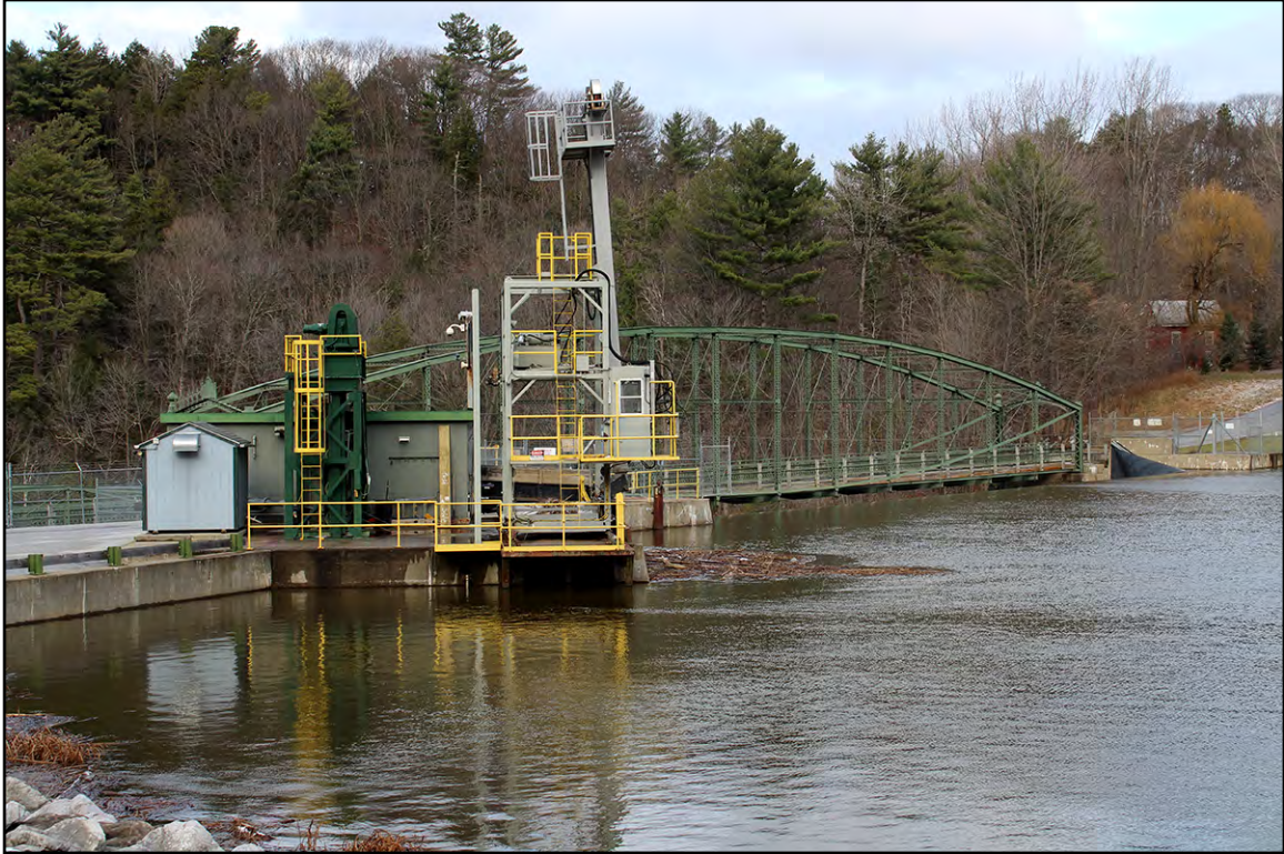
PLATE 4: Douglas & Jarvis Patent Parabolic Truss Iron Bridge, Crossing the Missisquoi River, Looking Northeast
