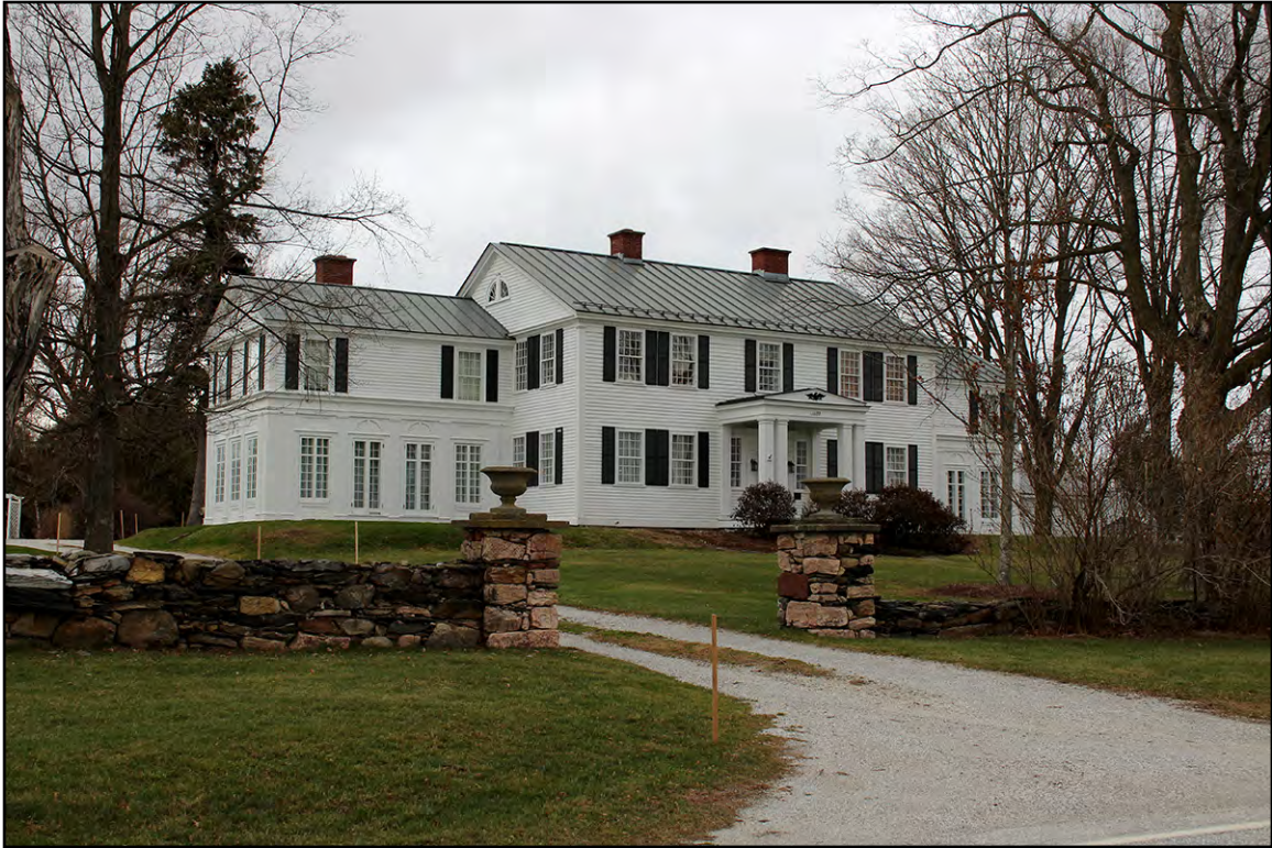
PLATE 8: Rockledge Farm, 2396 Highgate Road, Swanton, Looking Northwest
