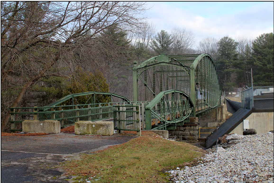
PLATE 5: Douglas & Jarvis Patent Parabolic Truss Iron Bridge, Crossing the Missisquoi River, Looking East
