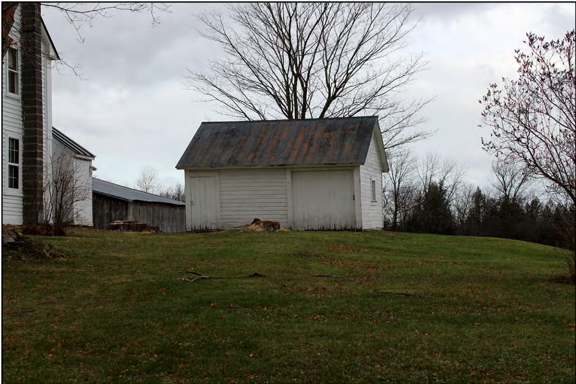
PLATE 16: Shed at Tarte House, 2384 Highgate Road, Swanton, Looking West
